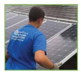
be fitted to either traditional roofs, flat roofs, walls or floor-mounted in the garden. The DC (Direct Current) electricity created is converted into usable power AC (Alternating Current) via a wall-mounted inverter in the attic. It then runs through a generation meter to be up and running well within a week of installation.
